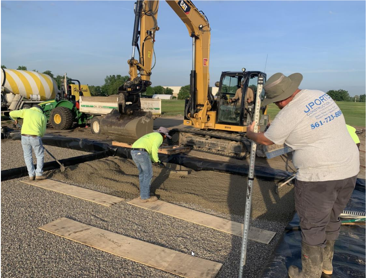
Figure 8. Capillary Concrete added to a depth of 5.08 cm, to provide a stable structure to the Capillary hydroponic system at the Capillary Hydroponic System and Variable Depth Rootzone research site at Michigan State University
