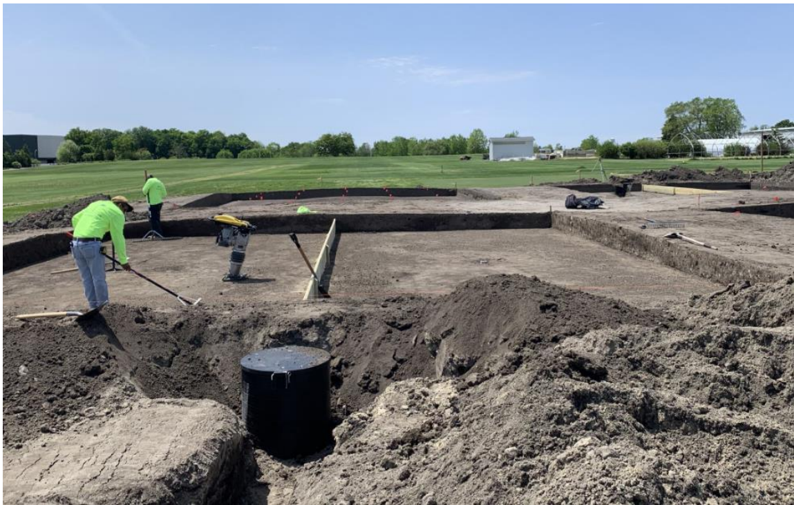
Figure 3. Control basin (foreground) installed adjacent to a Capillary Hydroponic System at the Capillary Hydroponic System and Variable Depth Rootzone research site at Michigan State University. The basin is aligned with the dividing board of the green cavity, and housing components that will transfer water in the green's cavity back and forth perpetually.
